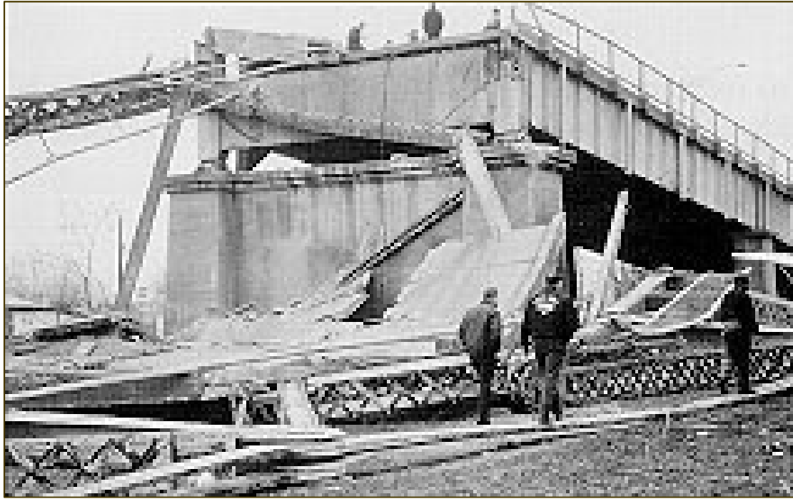
Collapsed in 1967, created awareness of “fracture critical components”
