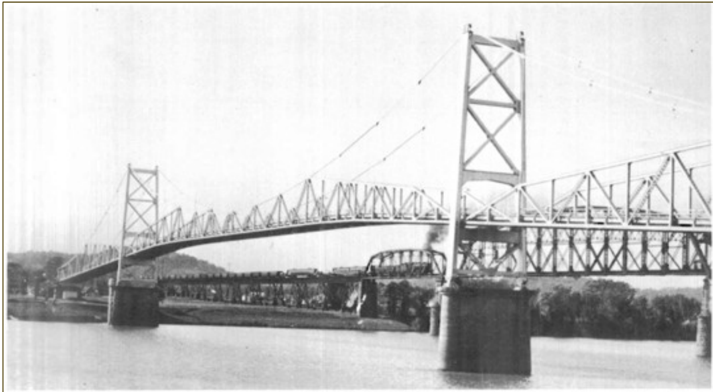
Silver Bridge on U.S. 35 in Ohio: Built 1924 Innovative optimization: High-strength steel 'eyebars' instead of cables
